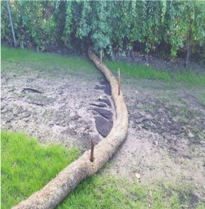
Fig 29: Erosion controls next to field house at UNH, north of the steam pipe. Viewing east. (8-29-19).
