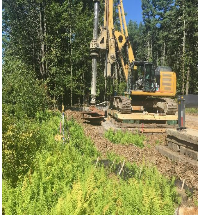
Fig 18: Prepping to drill Str. 100. Viewing west. (8-28-19).
