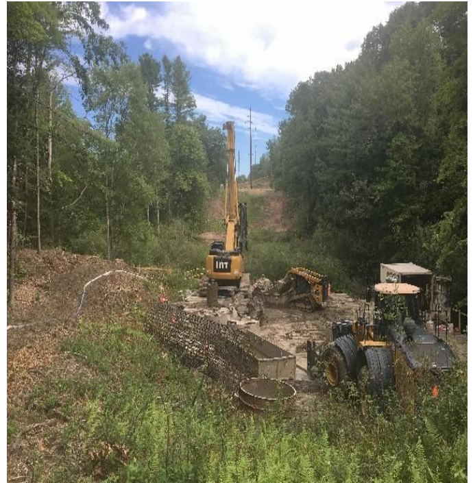
Fig 6: Drilling Str. 28 foundation. Viewing north. (8-23-19).
