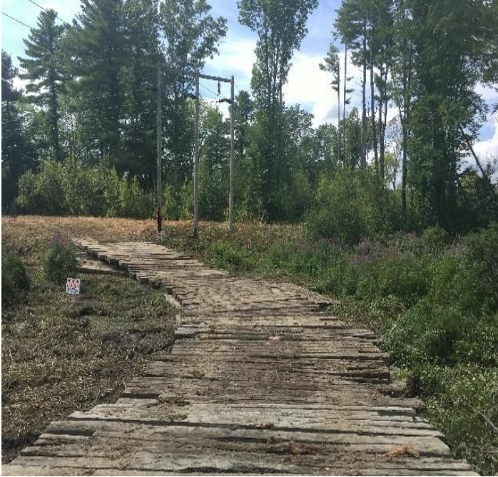
Fig 1: Wetland NW34 crossing. Viewing northwest. (8-22-19).
