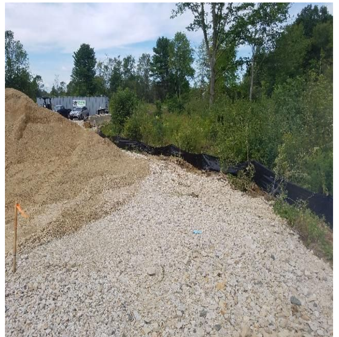
Fig 8: Siltation controls installed at Shattuck Rd laydown yard. Viewing west. (8-23-19).
