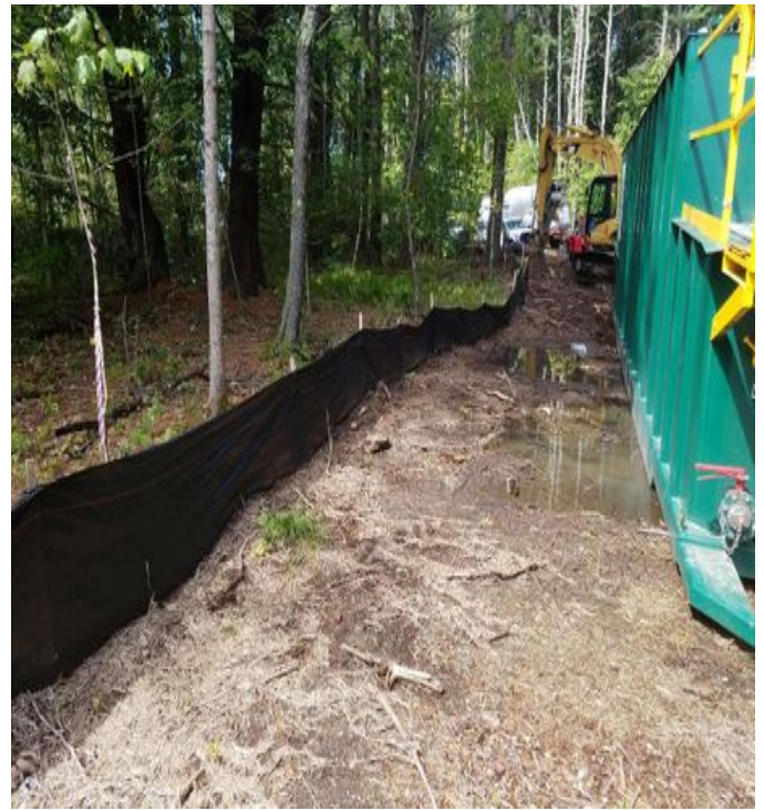
Fig 34: Repaired silt fence at Flynn Pit. Viewing west. (8-29-19).
