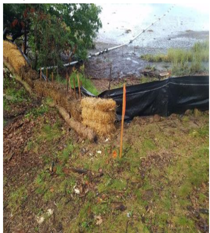
Fig 24: Erosion controls installed along Little Bay marsh. Viewing west. (8-29-19).
