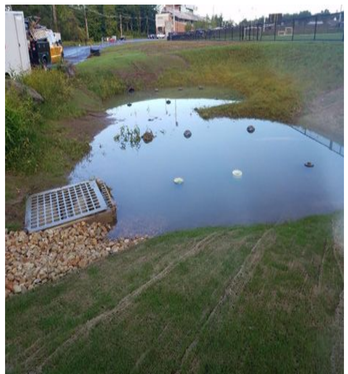
Fig 28: Rain garden at UNH. Viewing west. (8-29-19).
