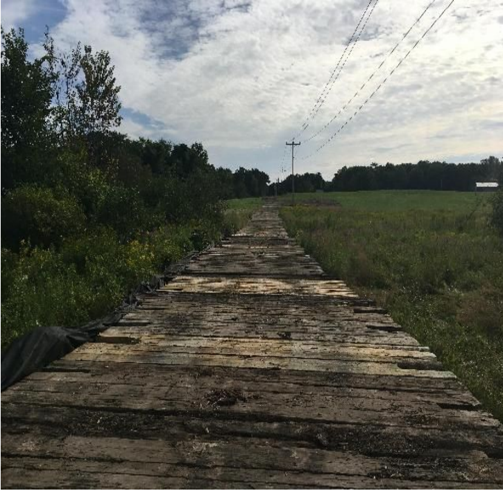
Fig 5: Wetland NW16 crossing. Viewing southeast. (8-23-19).
