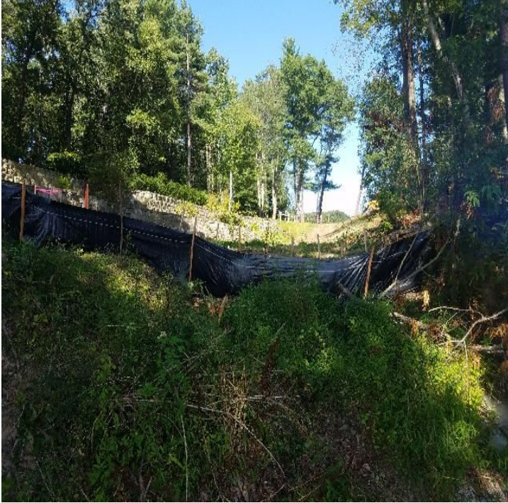
Fig 13: Erosion controls at Gundalow Landing. Viewing north. (8-26-19).
