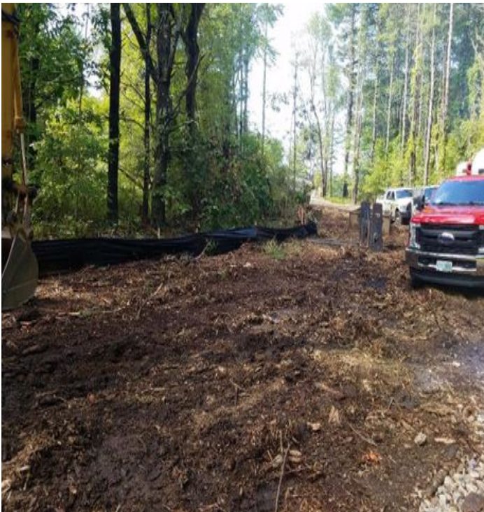
Fig 35: Repaired silt fence at Flynn Pit. Viewing west. (8-29-19).
