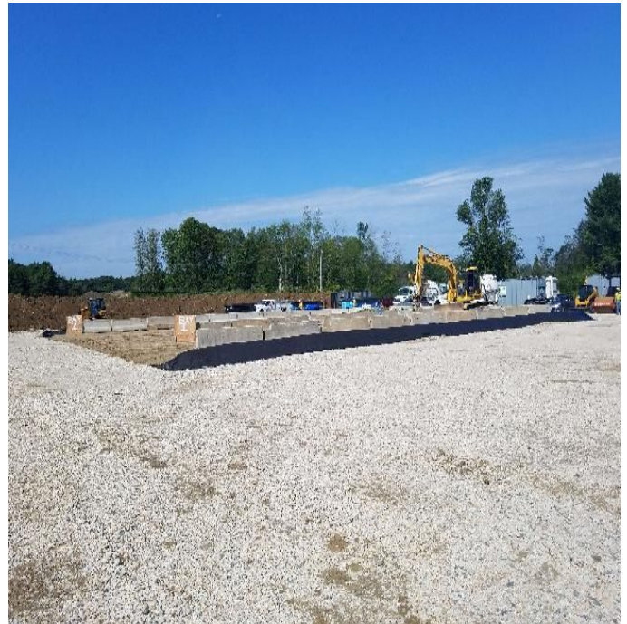
Fig 4 Shattuck Rd laydown yard progress. Viewing southwest. (8-22-19).
