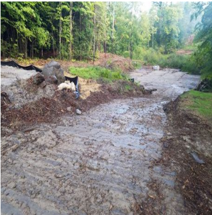
Fig 31: Sloped access down to Str. 28. Viewing north. (8-29-19).
