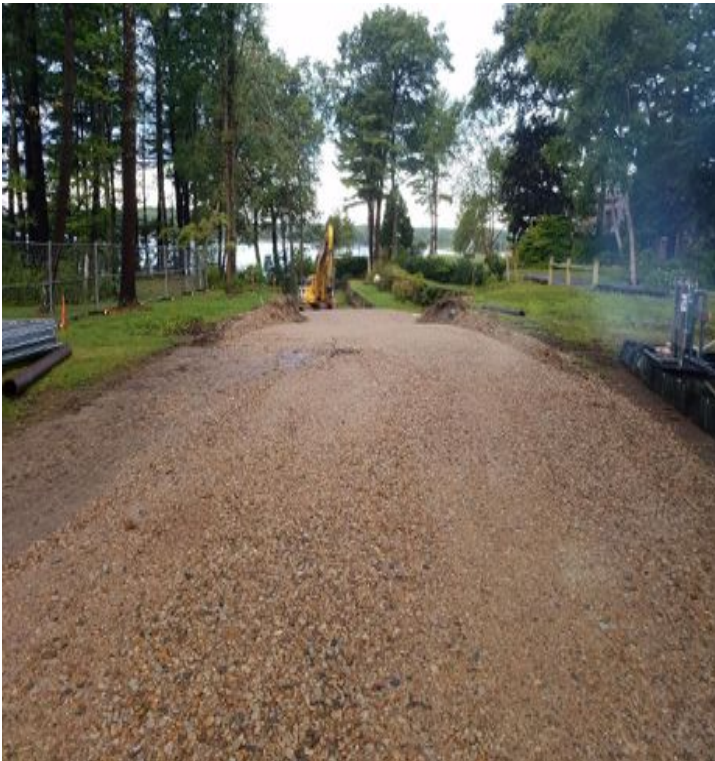
Fig 23: Access road at Gundalow Landing. Viewing west. (8-29-19).
