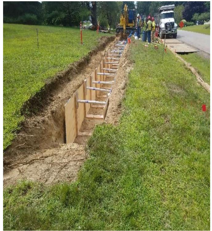
Fig 16: Trenching from Nimble Hill Rd into Gundalow Landing. Viewing west. (8-27-19).
