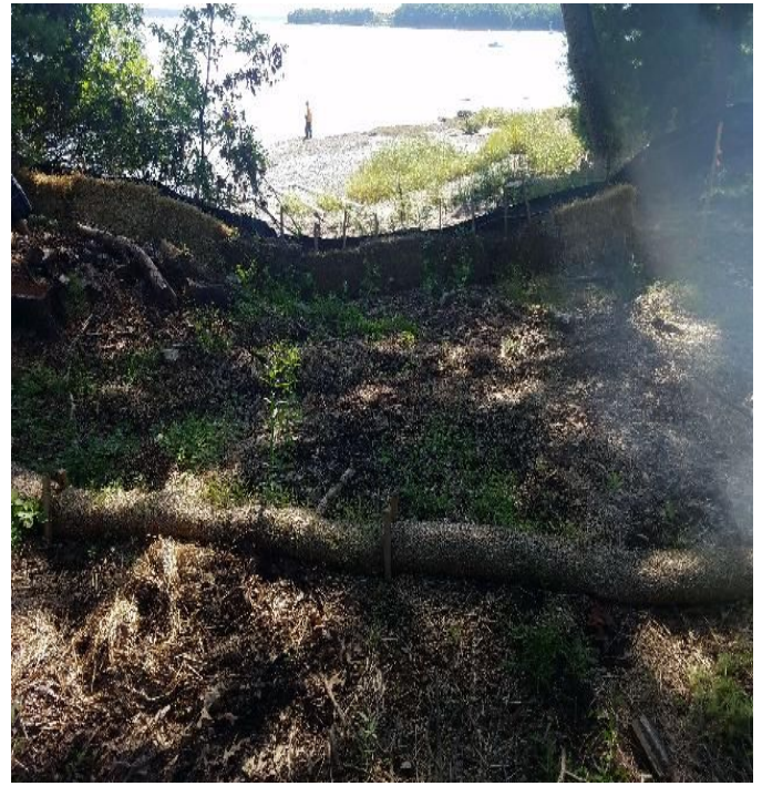
Fig 14: Erosion controls at Gundalow Landing. Viewing south. (8-26-19).
