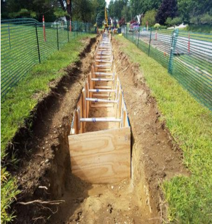
Fig 33: Trenching from Little Bay Rd to Gundalow Landing. Viewing west. (8-29-19).
