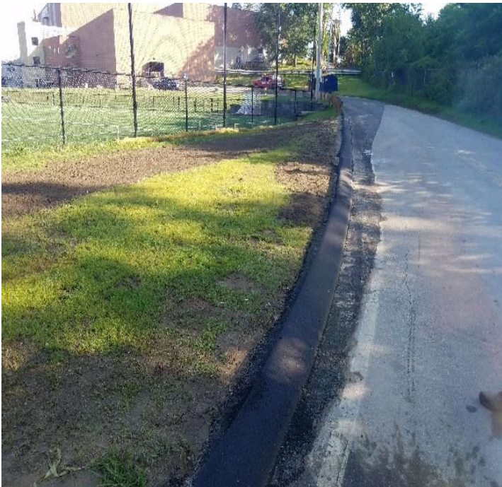
Fig 3: Restoration along Colovos Rd, UNH. Viewing north. (8-22-19).
