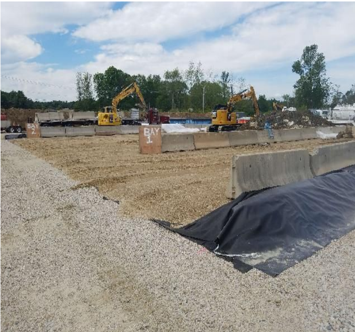
Fig 7: Shattuck Rd laydown yard progress. Viewing southwest. (8-23-19).
