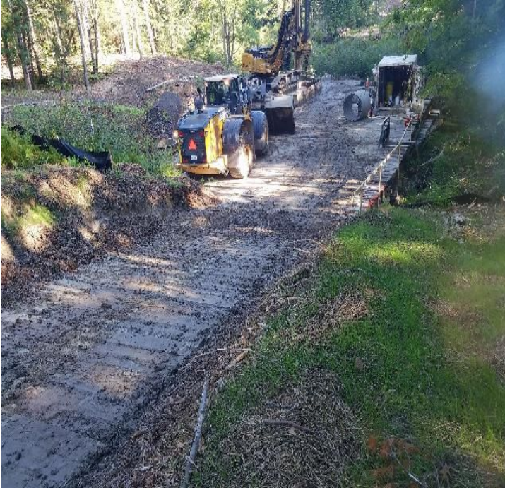
Fig 9: Drilling Str. 28 foundation. Viewing north. (8-24-19).
