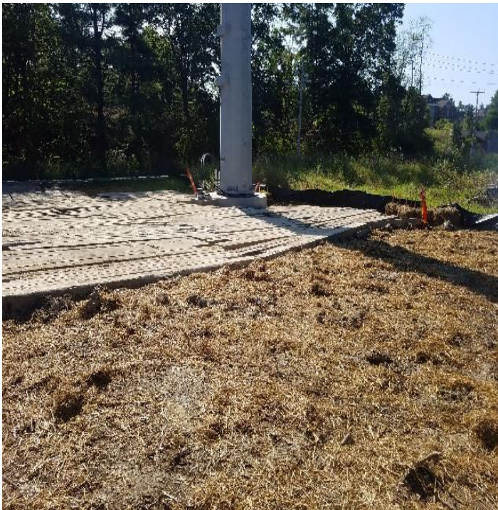
Fig 11: Str. 23 work site. Viewing southeast. (8-26-19).
